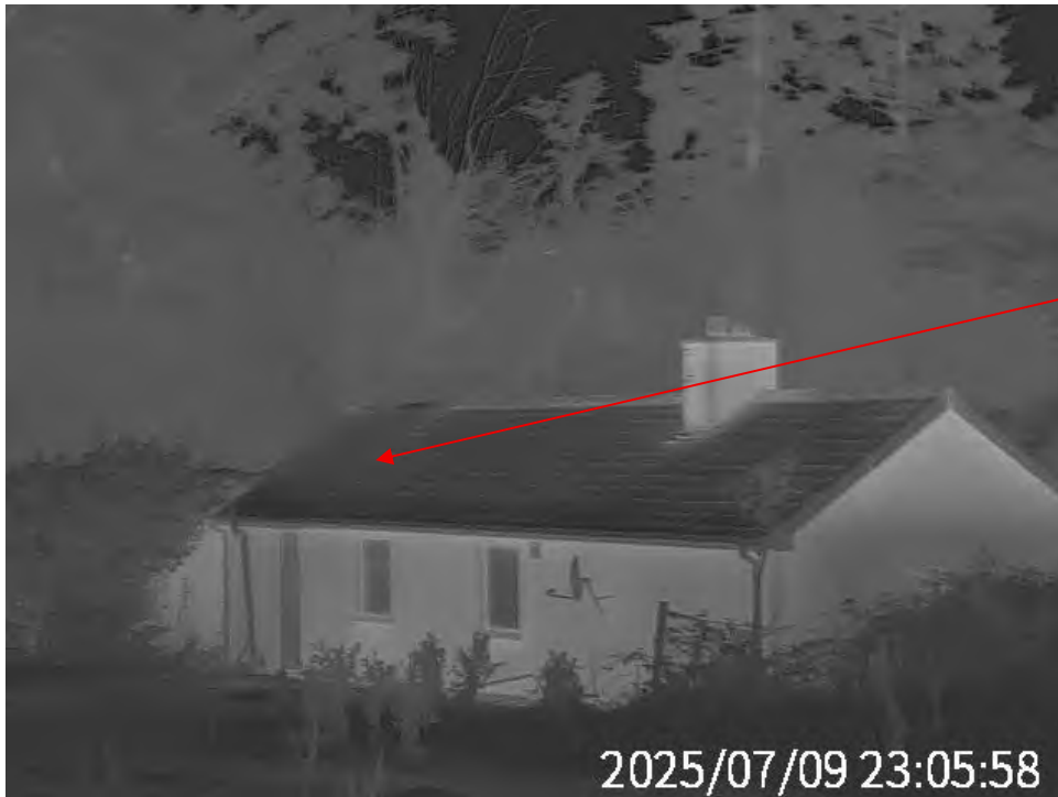
Photo 11 – thermal photo of rear of cottage. The point where single Soprano pipistrelle emerged from rear roof is indicated
