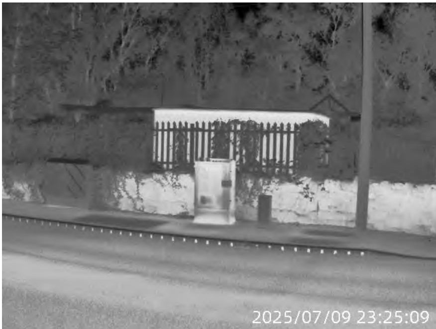
Photo 33 – southernmost building at pumping station
