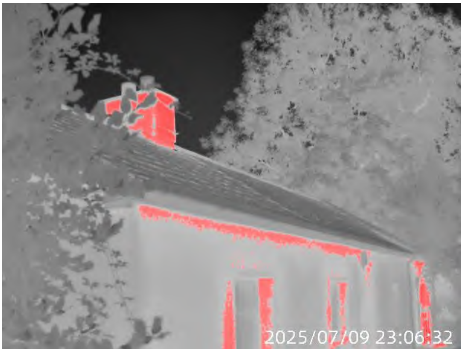
Photo 10 – thermal photo of front elevation of cottage
