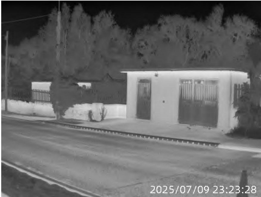
Photo 32 – northern most building at pumping station
