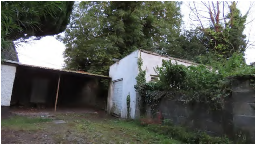
Photo 3 – shed attached to southern gable of cottage and garage to right hand side
