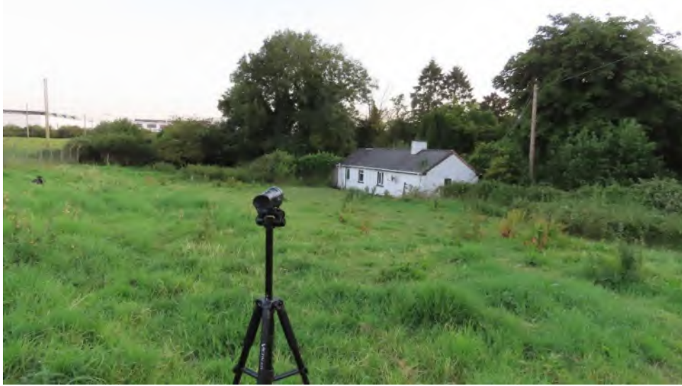
Photo 5 – Guide 19 thermal scope trained on rear elevation of cottage
