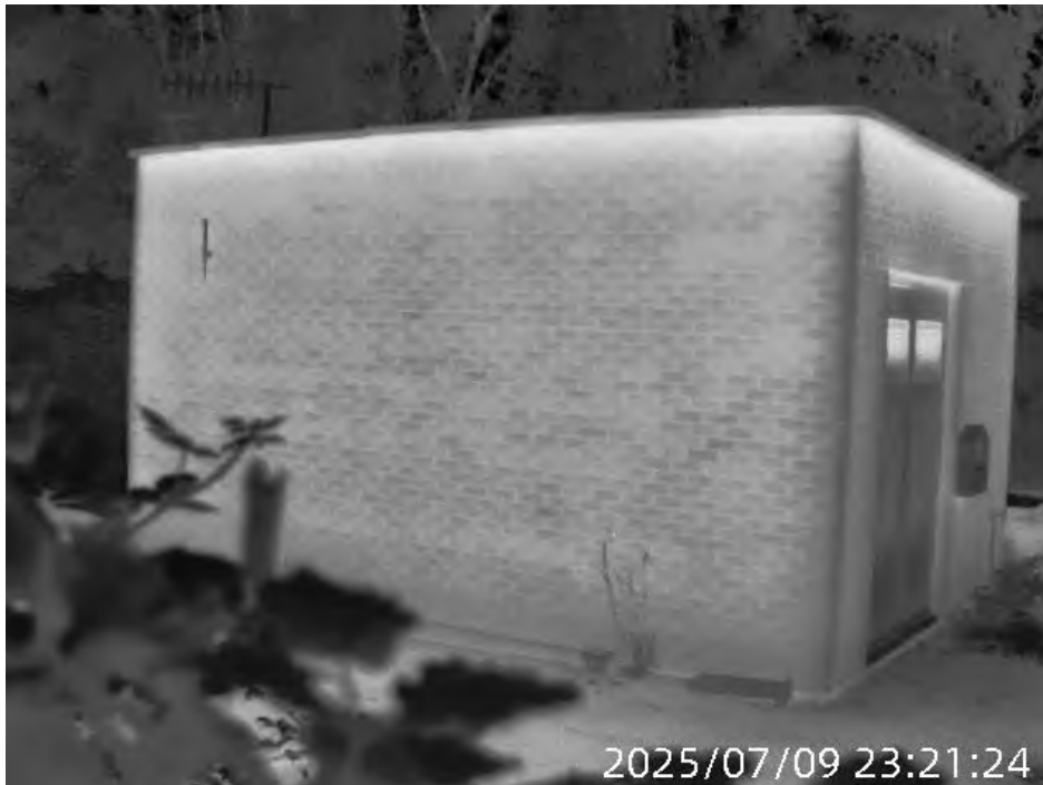
Photo 32 – thermal image of southernmost building at pumping station
