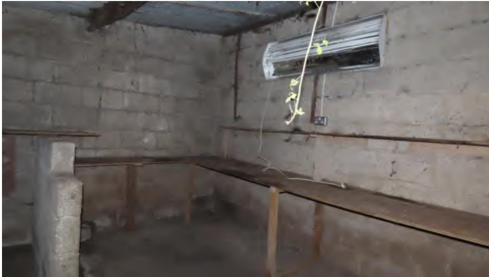
Photo 9 – interior of shed attached to cottage
