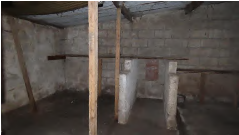
Photo 8 – interior of shed attached to cottage
