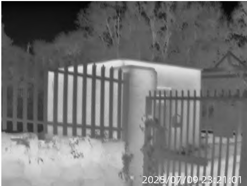
Photo 31 – thermal image of southernmost building at pumping station
